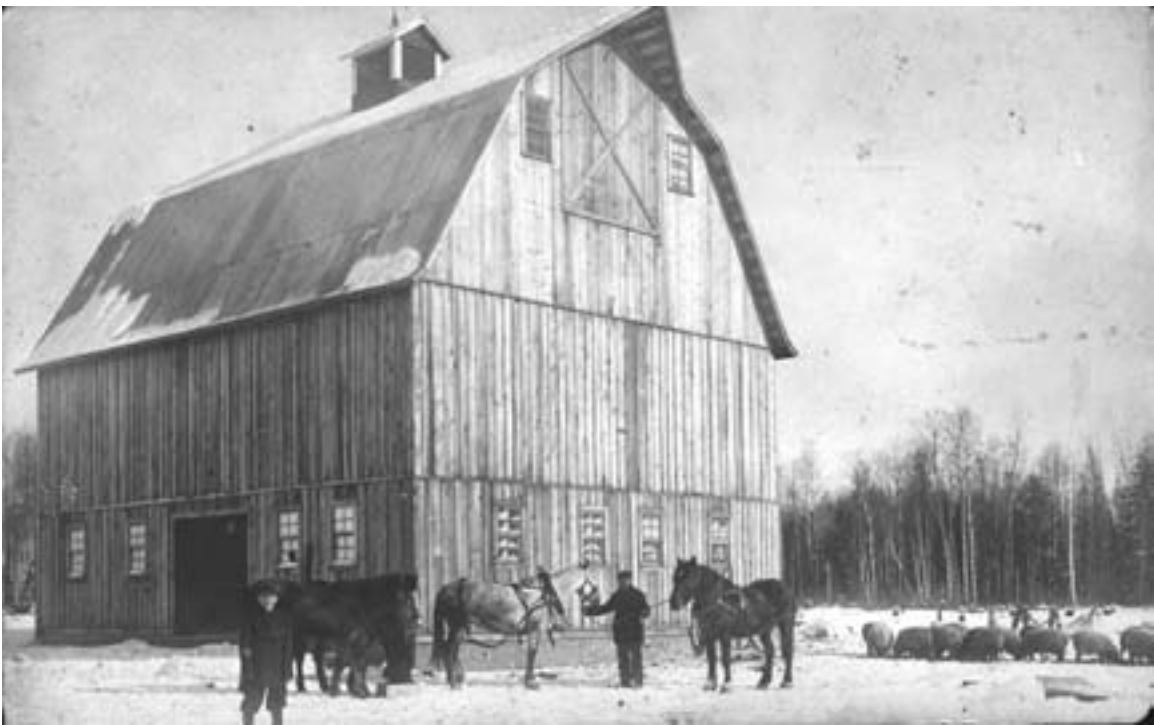
A barn sided with unpainted sawn lumber, probably in northern Minnesota. Location unknown, circa 1915. (MHS photo)
