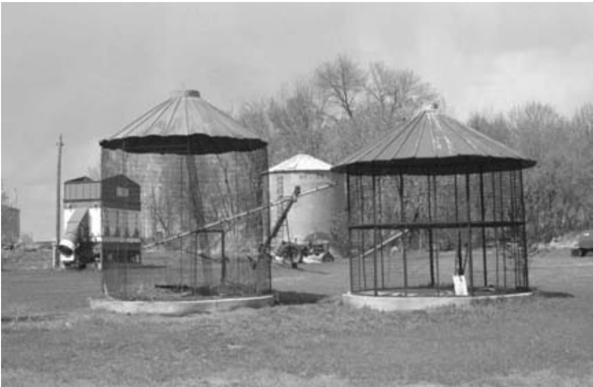
Two versions of prefabricated steel wire corncribs. Both have poured concrete floors and standing-seam metal roofs. Some cribs filled with ear corn can still be encountered in Minnesota. Stearns County, 2004. (Gemini Research photo)
