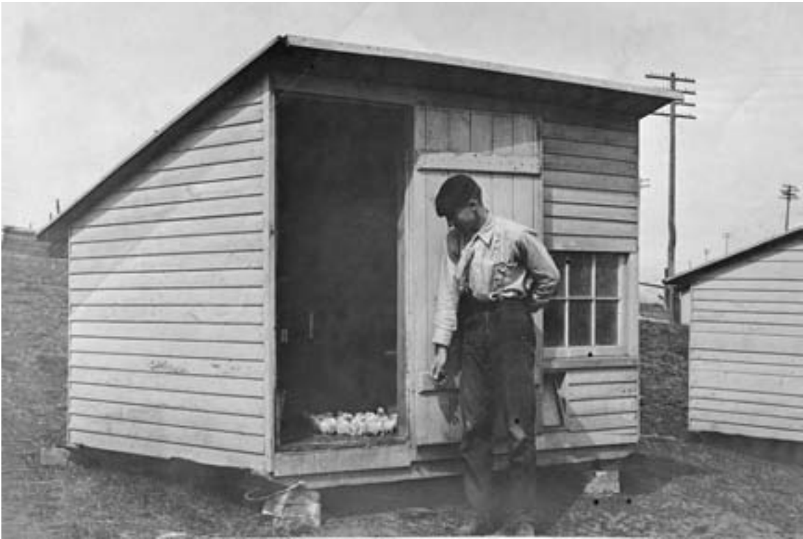
A colony brooder house with just-hatched chicks. Most brooder houses had little fixed equipment inside. An oil-, coal-, or electric-powered heater was needed for the first six to eight weeks to keep the chicks warm. Colony houses usually had temporary foundations, or were built on skids, so they could periodically be moved to fresh ground free of soil-harboring diseases. Location unknown, circa 1910. (MHS photo)
