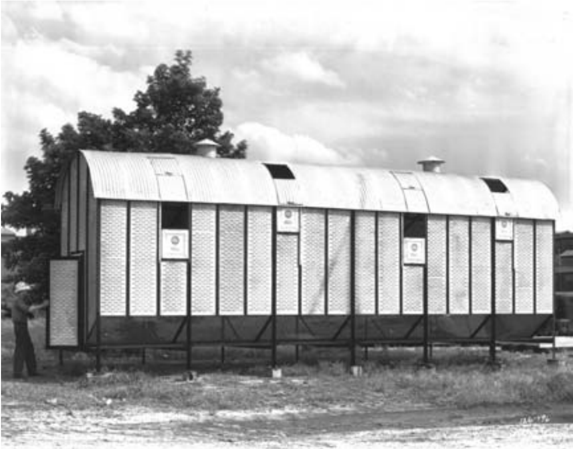
Prefabricated metal corncribs similar to this one were termed “experimental” in 1940 by Successful Farming magazine and the first models were just being marketed (Fox 1940). This version had perforated metal walls, which didn’t ventilate as well as walls of wire mesh. Location unknown, photo 1938. (MHS photo by Norton and Peel)
