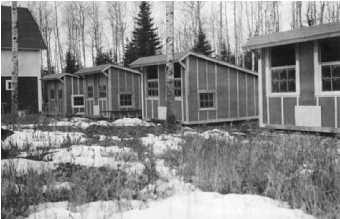
Colony brooder houses were used to raise chicks in small groups. Segregating the groups helped prevent the spread of parasites and disease, which were a serious problem. Because they required more materials and maintenance than a single structure, they were often used by farms raising large flocks and then only while the birds were young. The houses above appear to be sided with tar paper. Figreans Farm, St. Louis County, circa 1930. (MHS photo)
