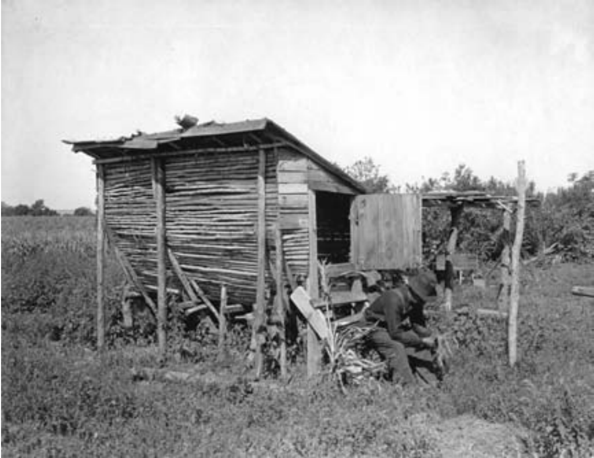
A single-pen corncrib of intricate pole construction. The man in the photo is shucking corn by hand. Location unknown, circa 1915. (MHS photo)
