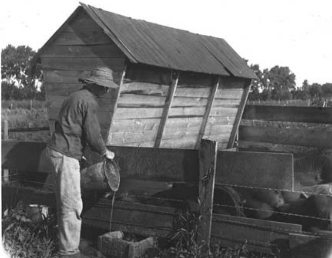
A single-pen, coffin- or keystone-style corncrib with walls and roof sheathed with planks. Location unknown, 1903. (MHS photo by Frank T. Wilson)
