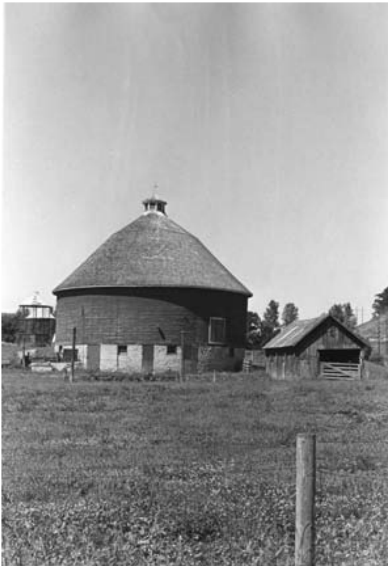
Round and other nonorthogonal barns were usually stall-type dairy barns. They sometimes had a central internal silo. Mount Vernon Township, Winona County, circa 1973. (MHS photo)
