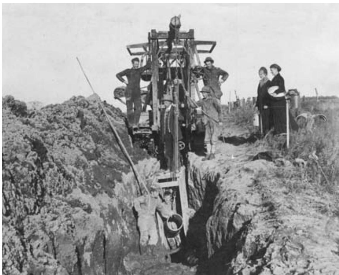
Laying subsurface drain tile with a machine. Shallow tiles and ditches were generally dug by hand. About four miles west of Dawson, Lac qui Parle County, circa 1905. (MHS photo)
