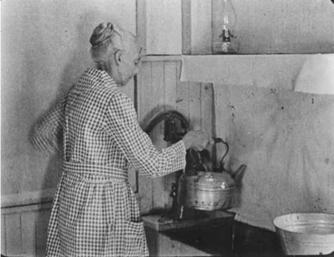
Hand-operated pitcher pumps were commonly used in farm kitchens to pump water from a cistern. The water was used for bathing and washing clothes and dishes. Location unknown, circa 1910. (MHS photo)
