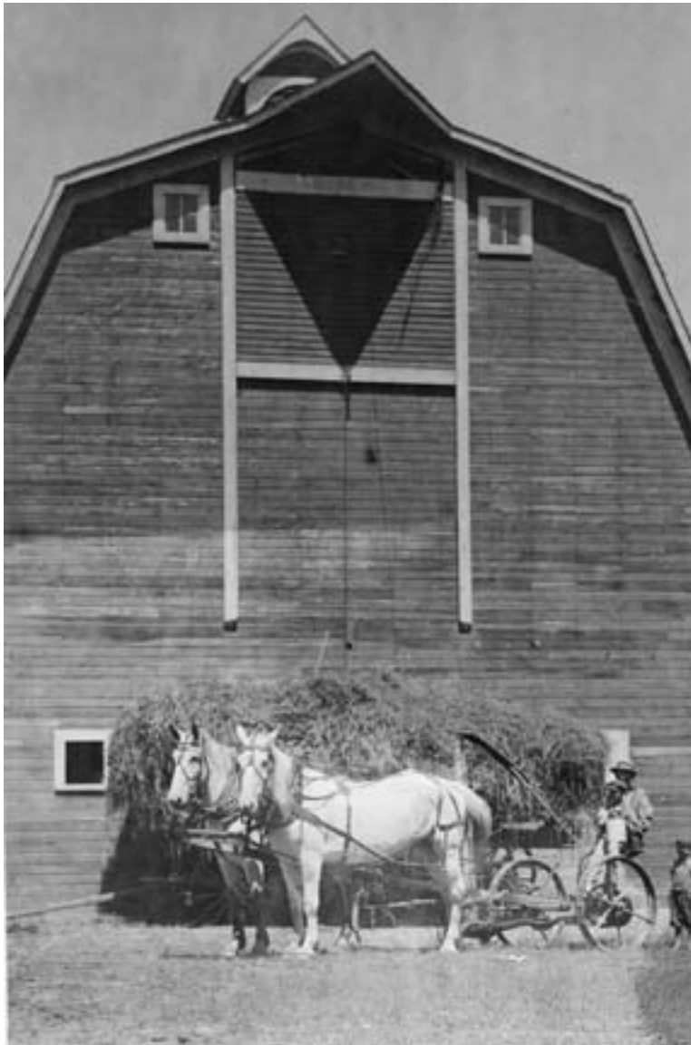
A load of hay ready for the loft. One Minnesota farmer in 1914 advised that the hay door be placed on the northern end of the barn so that the hot dusty chore of loading the hay in August could be done in the shade (Henry 1914). While second story lofts saved labor at feeding time, the dry hay was highly flammable and barn fires were common. Location unknown, circa 1910. (MHS photo by Harry Darius Ayer)
