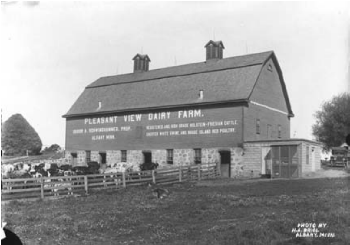
A dairy barn with stone basement and a concrete block milk house addition. The end walls feature decorative wood shingles, which is unusual. The painted lettering reads "Pleasant View Dairy Farm, Isidor A. Schwinghammer, prop., Albany, Minn., registered and high grade Holstein-Friesian cattle, Chester White swine, and Rhode Island Red poultry." Photo taken circa 1915. (MHS photo by Henry A. Briol)
