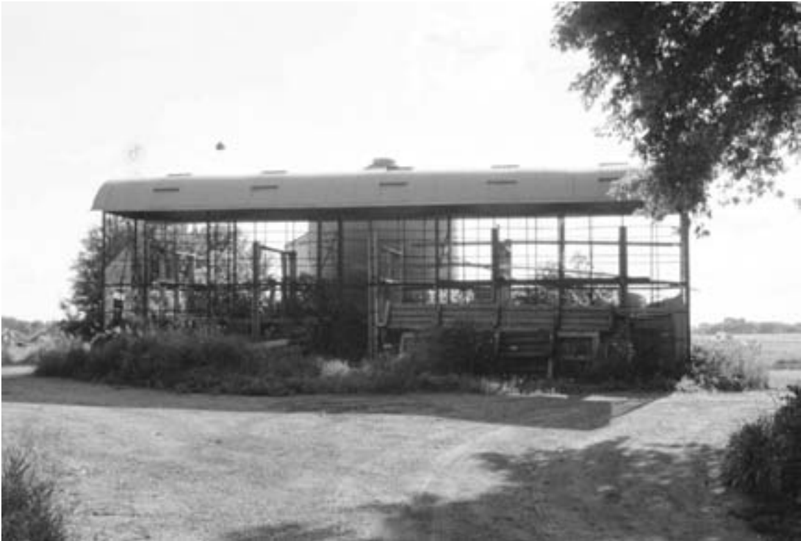
A steel wire corncrib now used for miscellaneous equipment storage. McLeod County, 2003. (Gemini Research photo)
