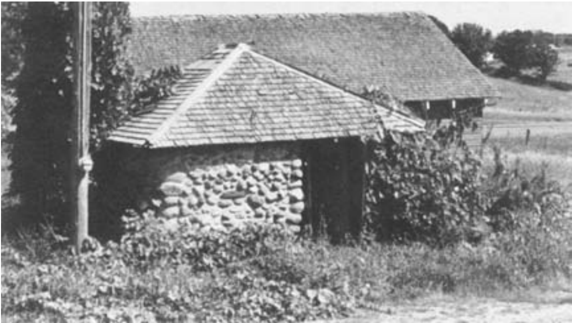
This fieldstone springhouse was standing in Mille Lacs County in the early 1980s. It was built into the side of a slope, which was typical. From Brinkman and Morgan's Light from the Hearth: Central Minnesota Pioneers and Early Architecture (1982).
