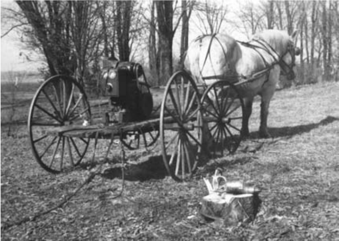
It was common on Minnesota farms to use a gasoline-powered generator to produce electricity for lighting, and to move the gasoline engine around the farm to power equipment that would saw wood, separate cream, sharpen tools, or wash clothes. Location unknown, circa 1925. (MHS photo)
