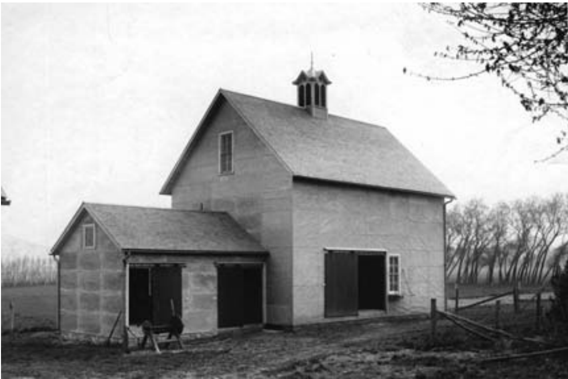
A power house (left), grinding tool (front), and granary (right). Both buildings were covered with pressed metal siding simulating brickwork. Location unknown, circa 1910. (MHS photo by Harry Darius Ayer)
