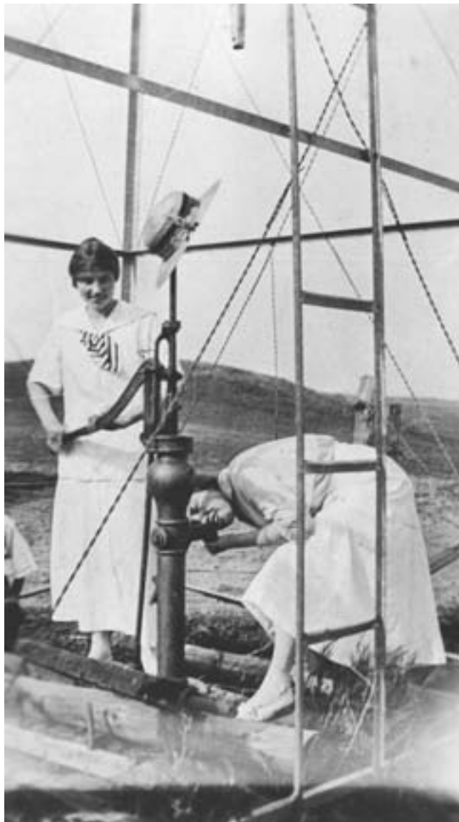
A hand-operated well pump at the base of a steel windmill tower. Photo taken near Nassau in Lac qui Parle County, circa 1912. (MHS photo)
