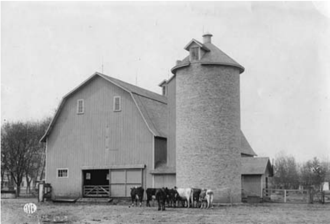
Brick silos were first built around the turn of the century. They were expensive to construct and, like all silos built of masonry units, had to be lined with a coating of concrete to protect the mortar from the corrosive silage. Henry Farm, location unknown, circa 1910. (MHS photo by Harry Darius Ayer)
