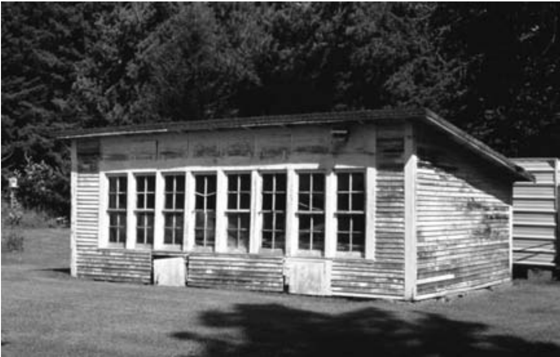
A 12' x 18' poultry house like this one would only be suitable for a small flock of about 60 chickens. Built circa 1924, this house has clapboard siding, eight double-hung windows, and a pedestrian door in the end wall. Its shed roof is covered with rolled asphalt roofing. Scott Farm, Garrison Township, Crow Wing County, 2003. (Gemini Research photo)
