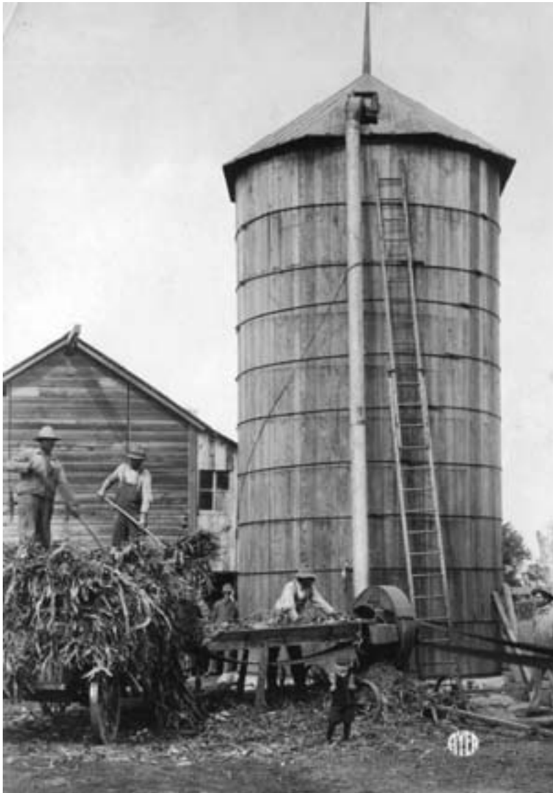
Vertical stave silos, first built in the 1890s, were easier to construct than those of horizontal wood and became more popular. The tongue-and-groove staves were reinforced with iron bands whose turnbuckles were periodically tightened. Note the belt-operated silo filler and the lightning rod on the silo roof. Location unknown, circa 1910. (MHS photo by Harry Darius Ayer)
