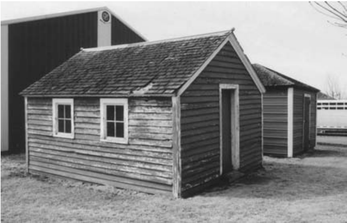
This summer kitchen may date from about 1930. It had a simple design with three windows for ventilation. A stove (removed) stood against the rear wall (opposite the door), with the stove pipe projecting through the roof. Anderson Farm, Stevens County, 2005. (Gemini Research photo)
