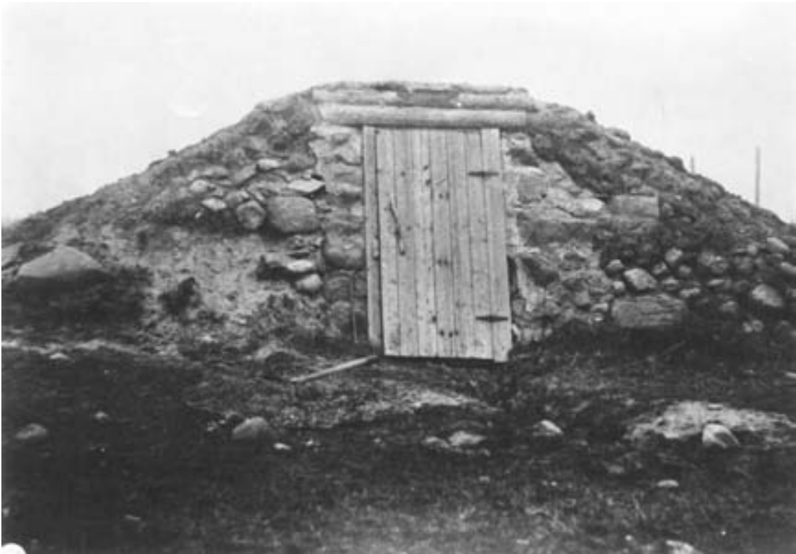
Many root cellars were built of stone rubble. Some were dug into hillsides; others were partly excavated and then banked with earth and sod. Konristo Farm, Carlton County, 1918. (MHS photo by St. Paul Dispatch )
