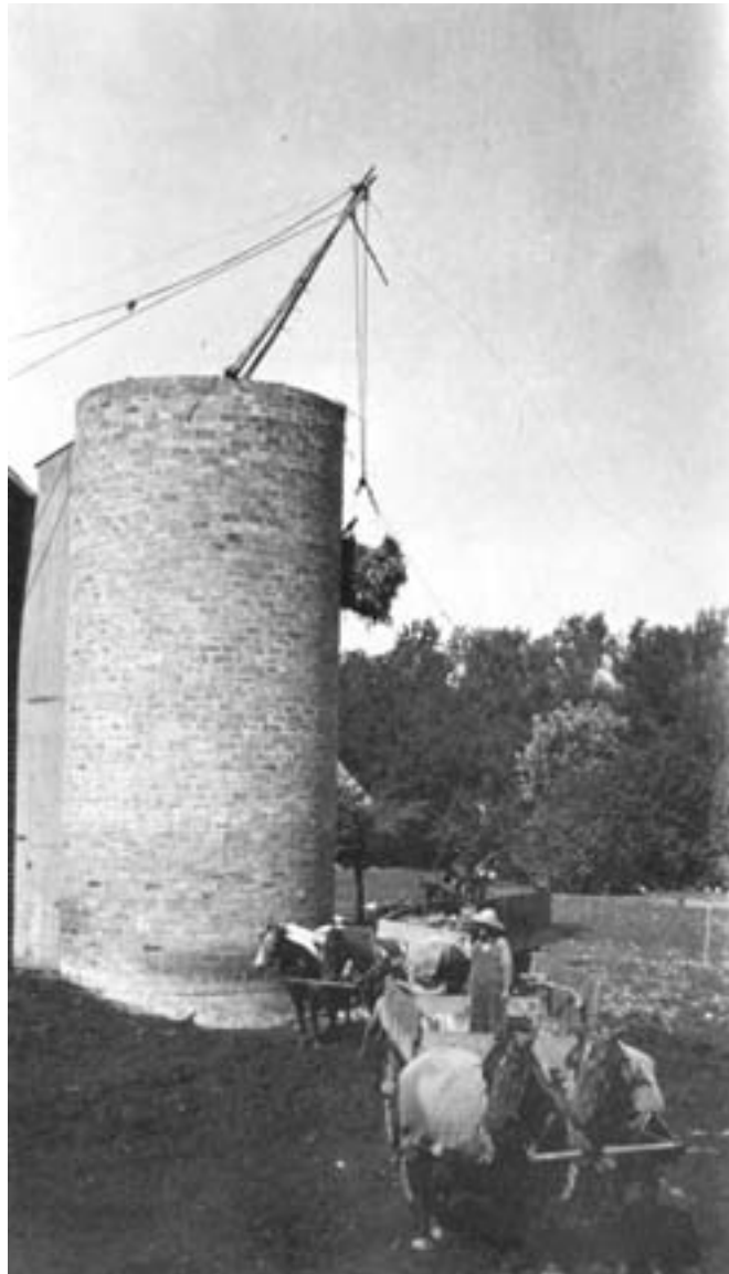
Silos were becoming common in Minnesota around 1910, and by 1927 the state had one silo for every five farms. The farmers in this photo are filling a silo with a sling system. Ronning Farm, Lac qui Parle County, circa 1915. (MHS photo)
