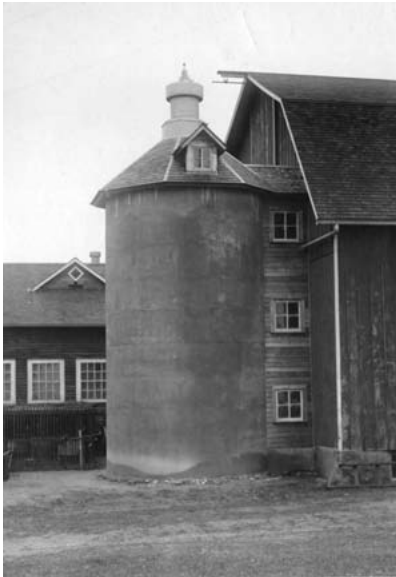
Reinforced concrete silos were built in layers by moving the forms successively upward. Like most silos, this one was attached to the barn. Location unknown, circa 1910. (MHS photo by Harry Darius Ayer)
