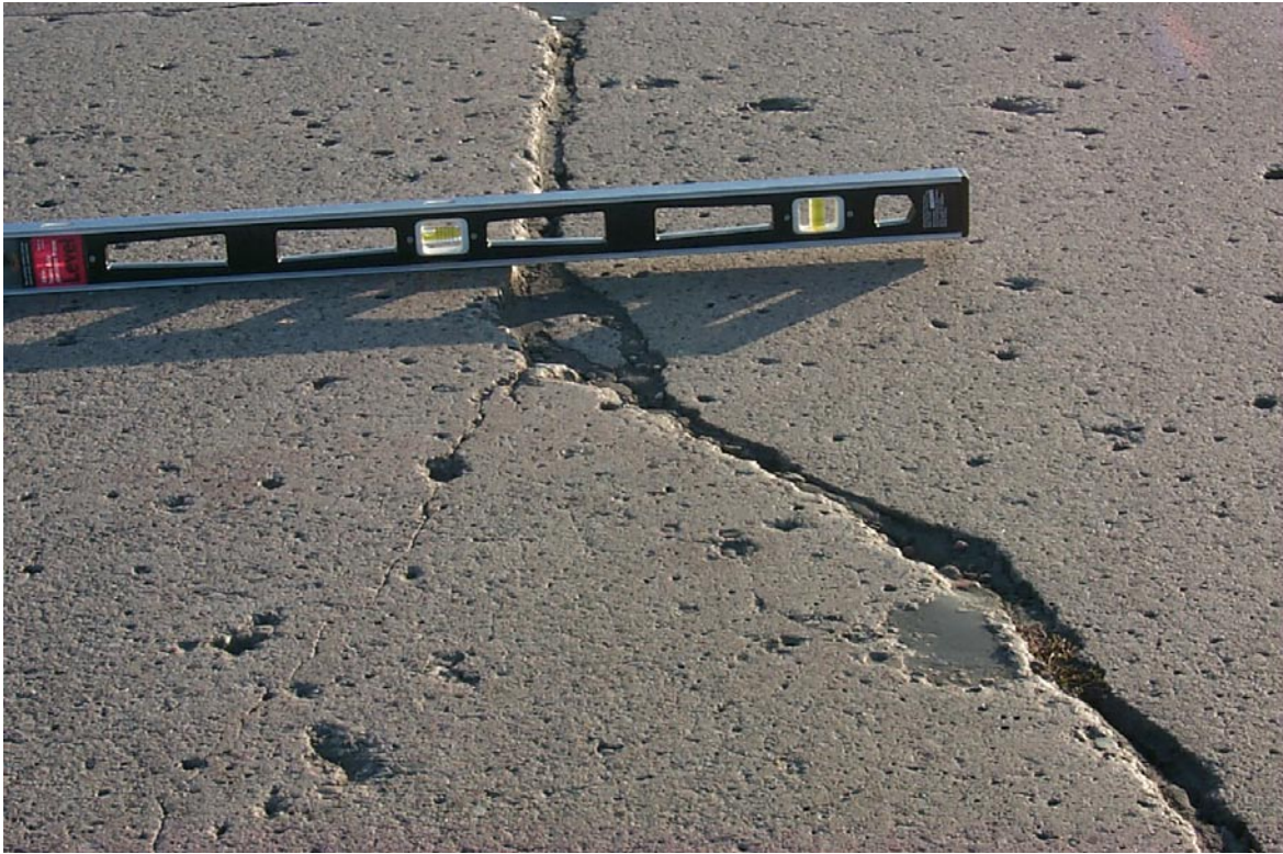
Figure 39. Faulted Panel
