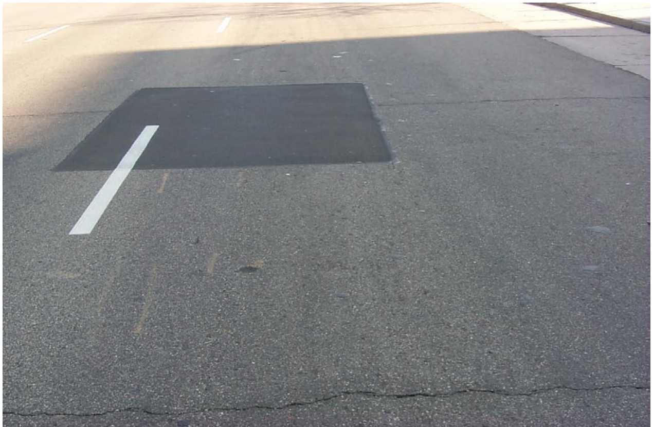
Figure 24. Bituminous Patching
