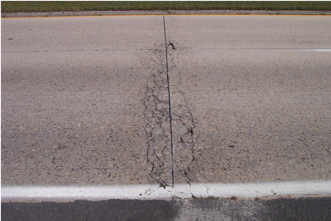
Figure 43. D-Cracking
