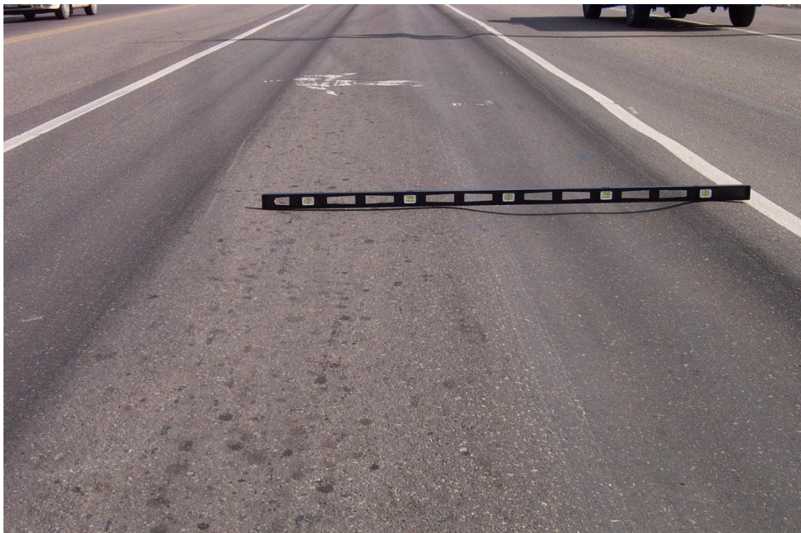
Figure 22. Rutting (0.50 inches or greater)
