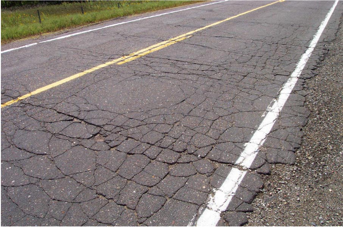
Figure 21. Alligator Cracking
