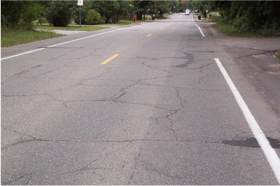
Figure 18. Multiple Cracking
