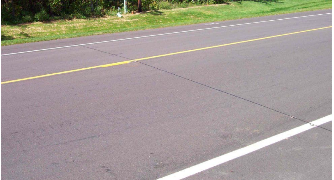
Figure 3. Low Severity Transverse - Saw and Seal
