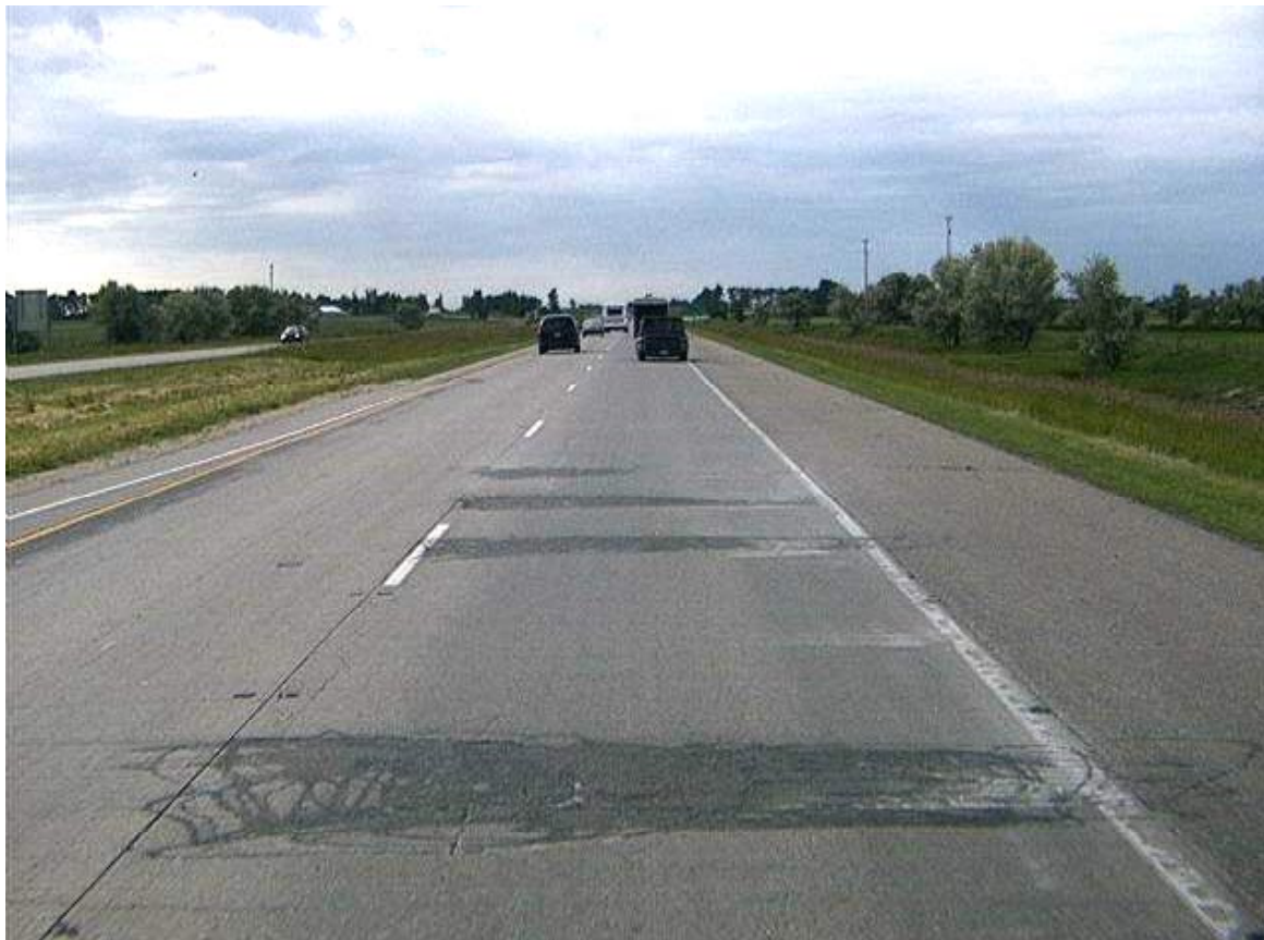
Figure 44. Patch Deterioration
