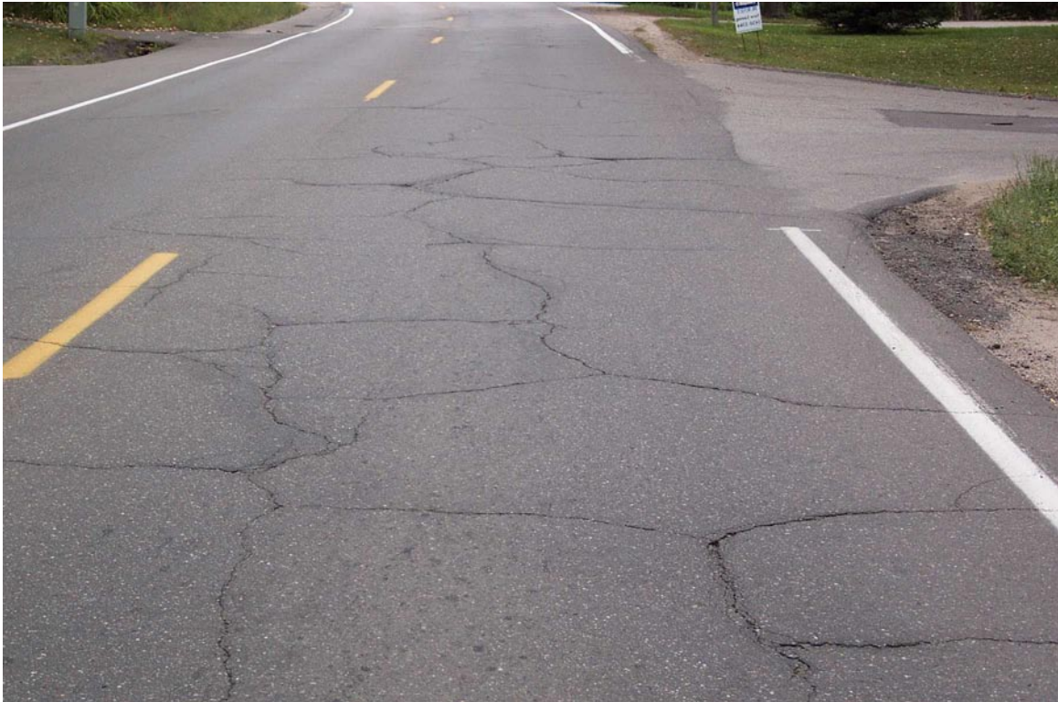
Figure 17. Multiple Cracking
