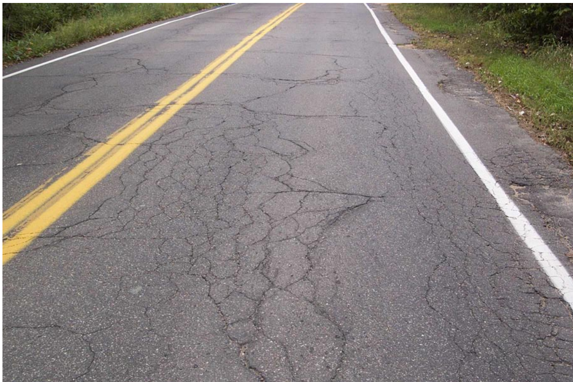
Figure 20. Alligator Cracking
