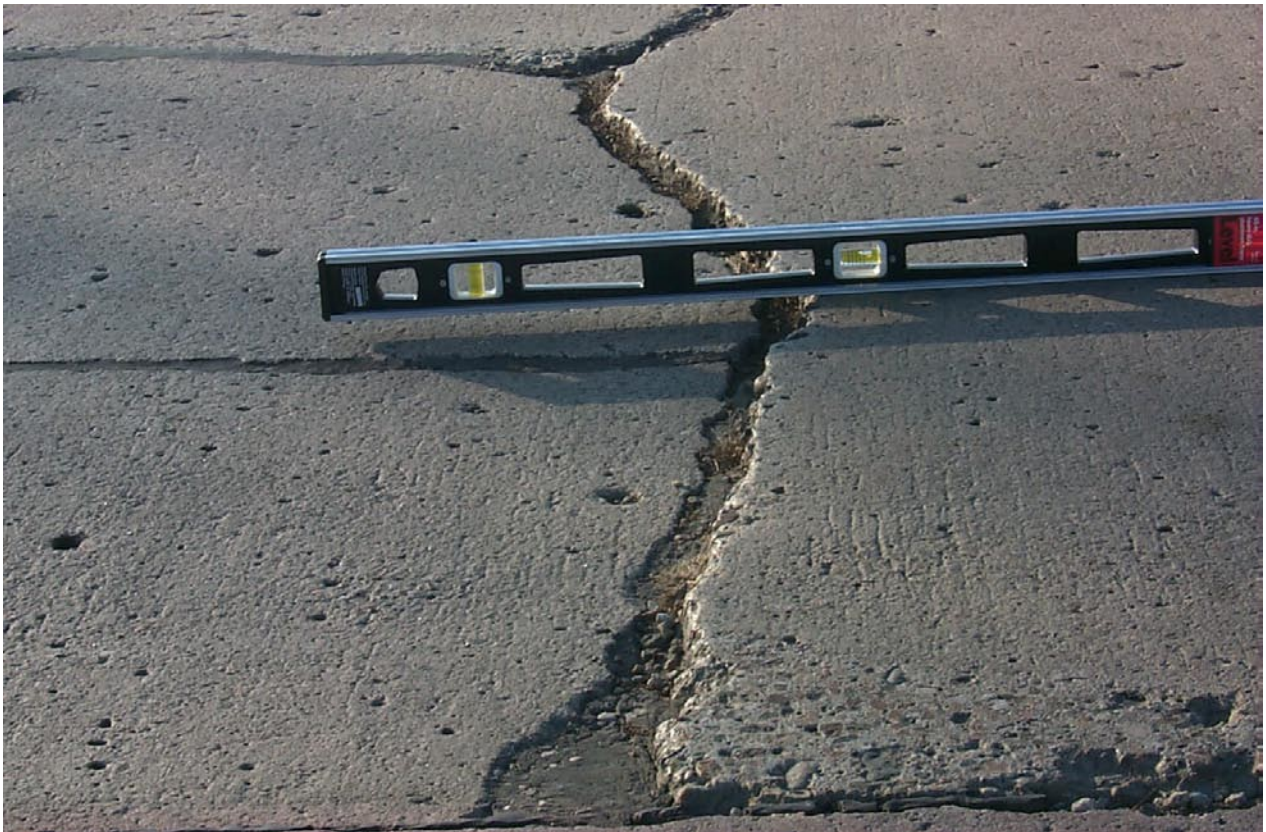
Figure 37. Faulted Panel
