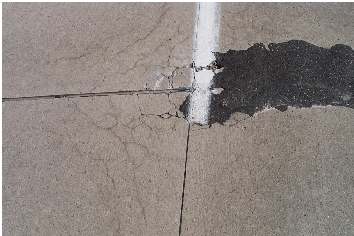
Figure 46. D-Cracking
