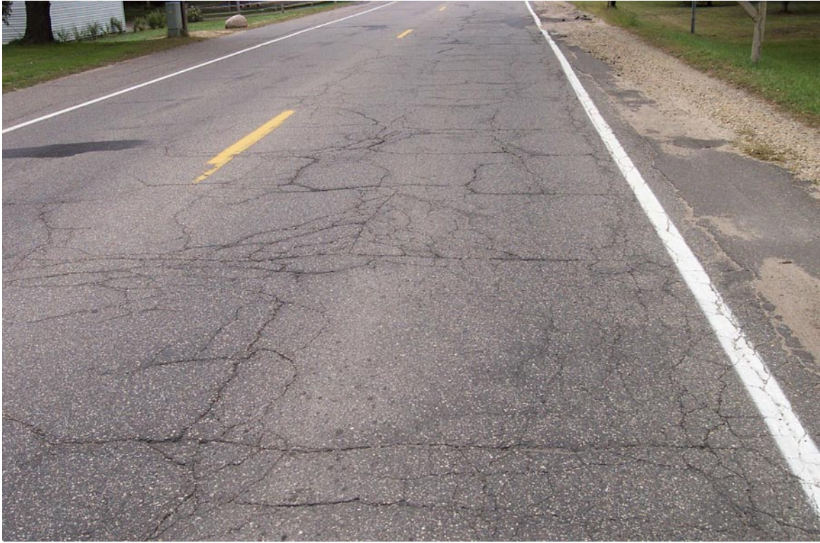
Figure 19. Multiple Cracking
