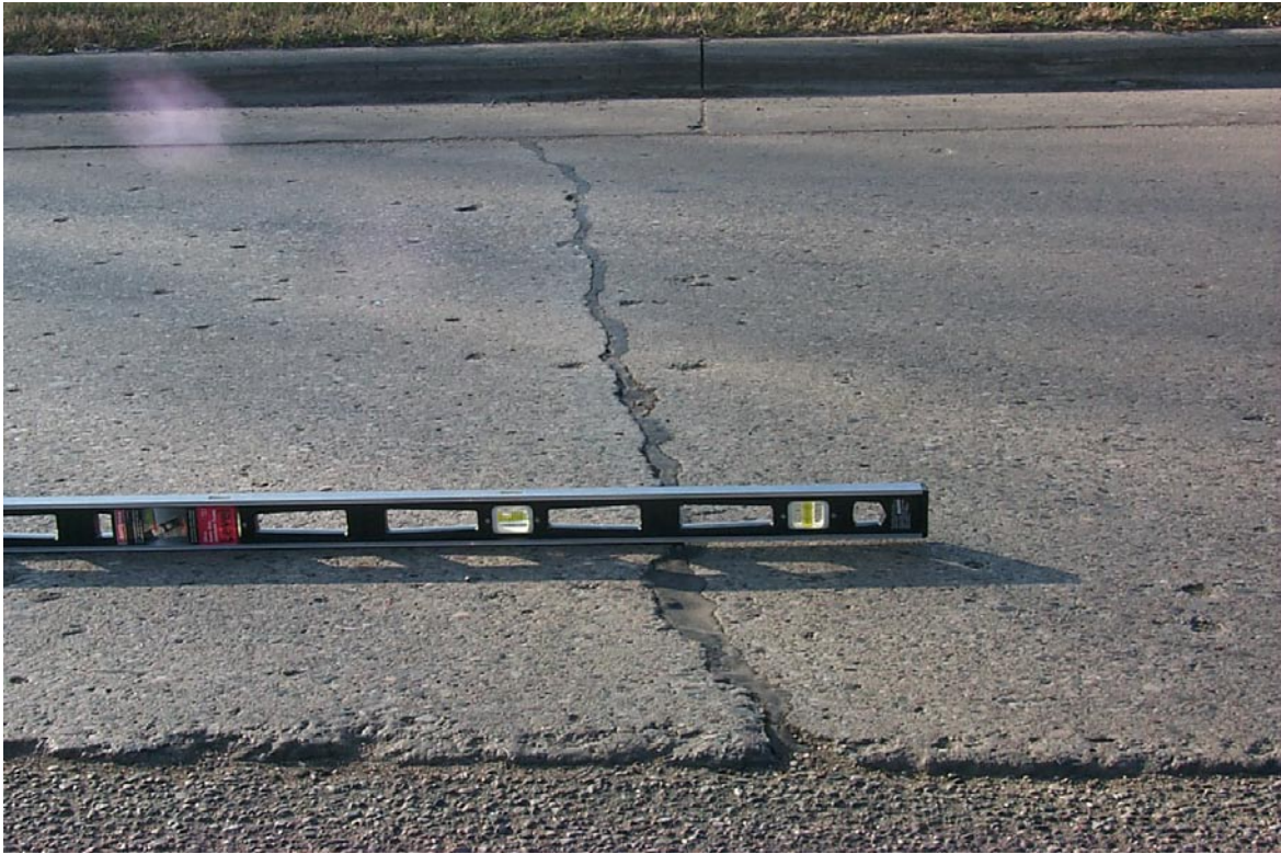
Figure 38. Faulted Panel
