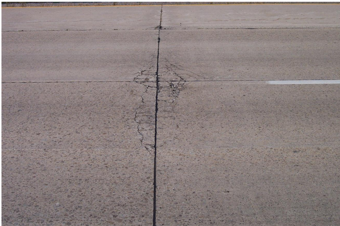
Figure 41. D-Cracking
