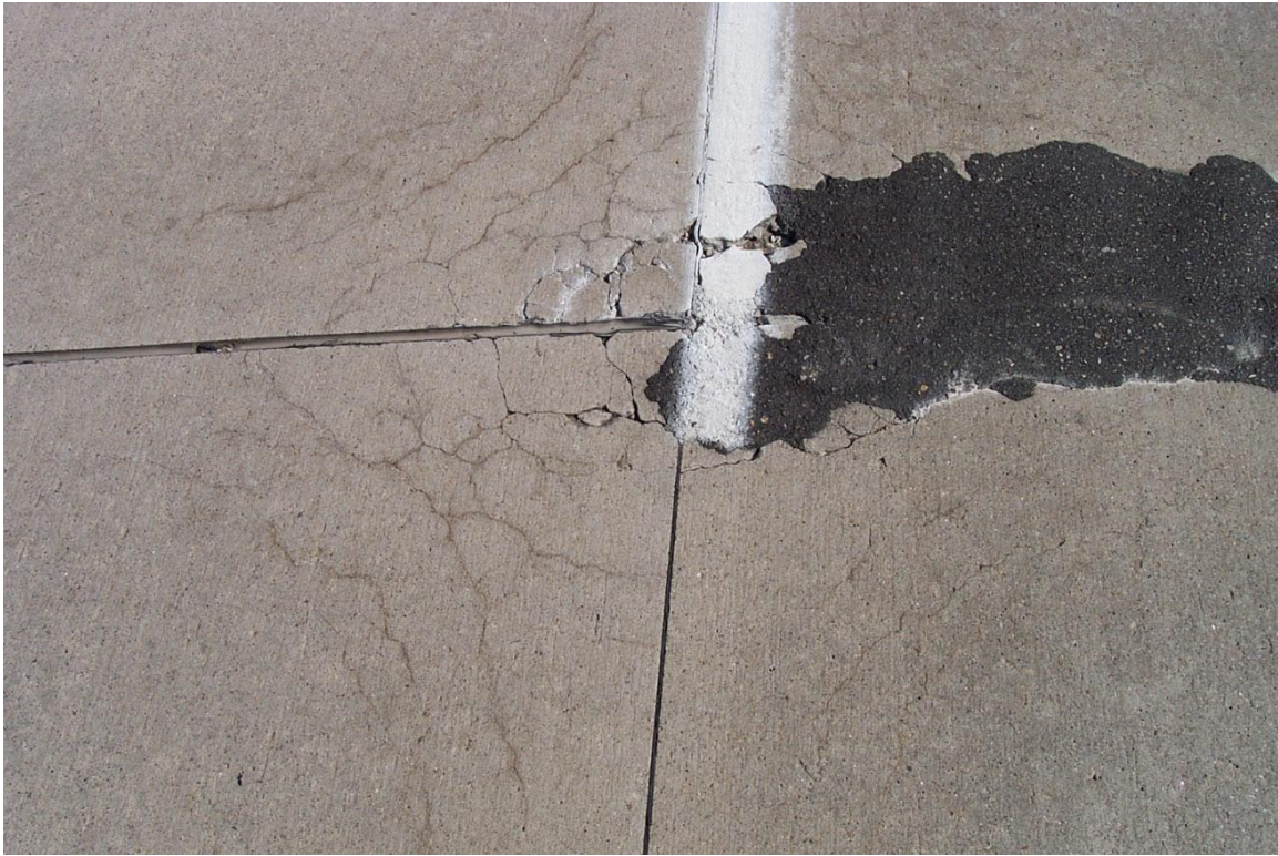
Figure 42. D-Cracking
