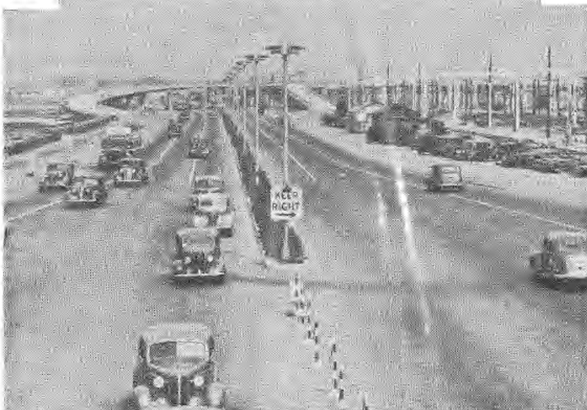
Division of the Eastshore Highway approach to the San Francisco-Oakland Bay Bridge with a median strip was the Bay Region's most important recent contribution toward the cause of accident prevention, in the opinion of traffic experts. The result has been a minimum of collisions on one of the most heavily traveled thoroughfares in Northern California.
