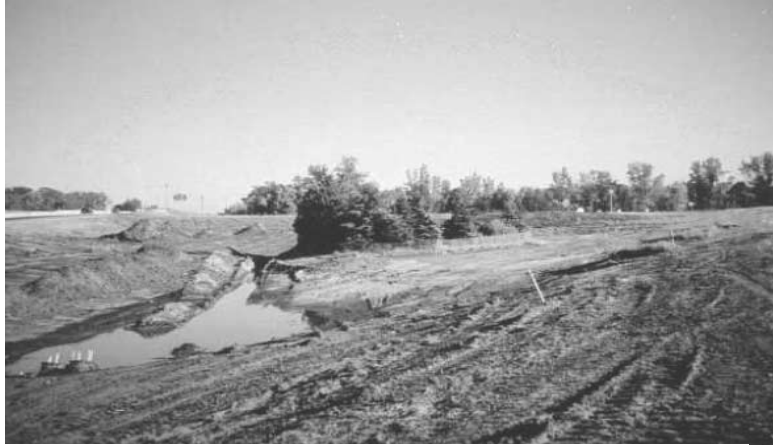
Figure 9-12. Protecting Trees during Construction
