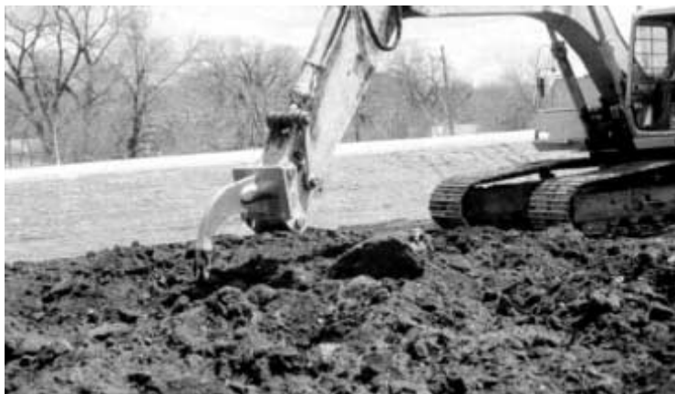
Figure 9-10. Scarifying the Soil - during construction significantly improves the chances of any vegetation establishment.
