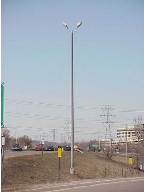
Double Vertical Mount Pole Arrangement (VMD-45)
