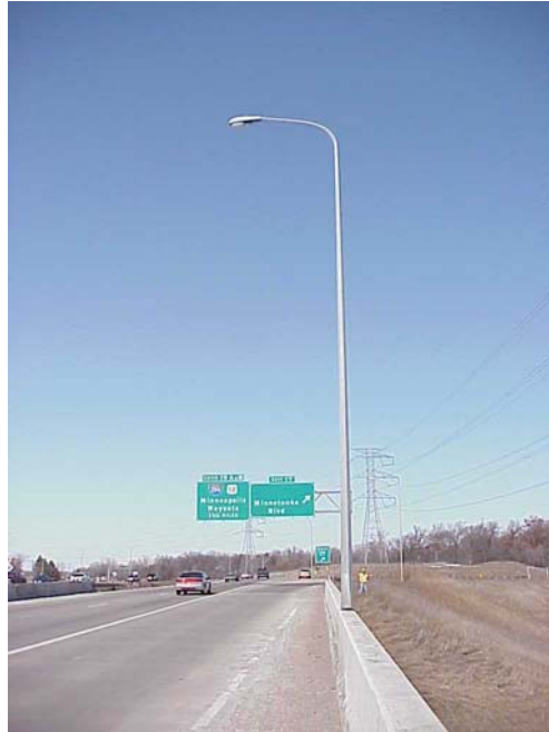
Bridge Pole (6B-40)
