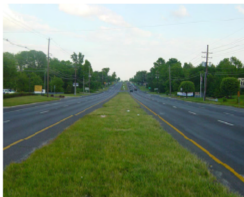
Route 73 in Burlington County is the prototypical regional arterial in a suburban setting, with divided median and wide shoulders.
