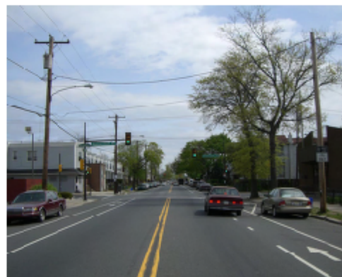
Torresdale Avenue in Philadelphia, which functions as a community collector in an urban area, has 11 ft. travel lanes, 5 ft. bike lanes, 8 ft. parking lanes, and 6 ft. sidewalks.
