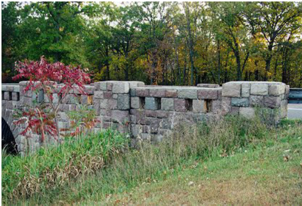
10. North End of East Wall looking Southwest
