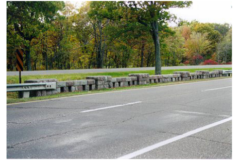
3. View of West Wall across TH 169—looking NW
