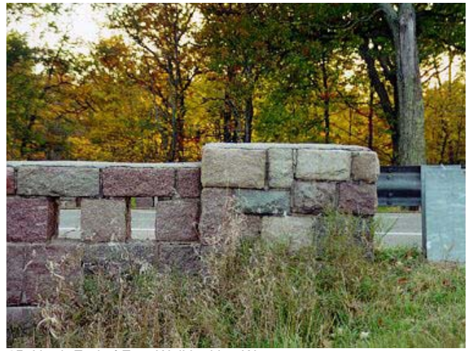
15. North End of East Wall looking West
