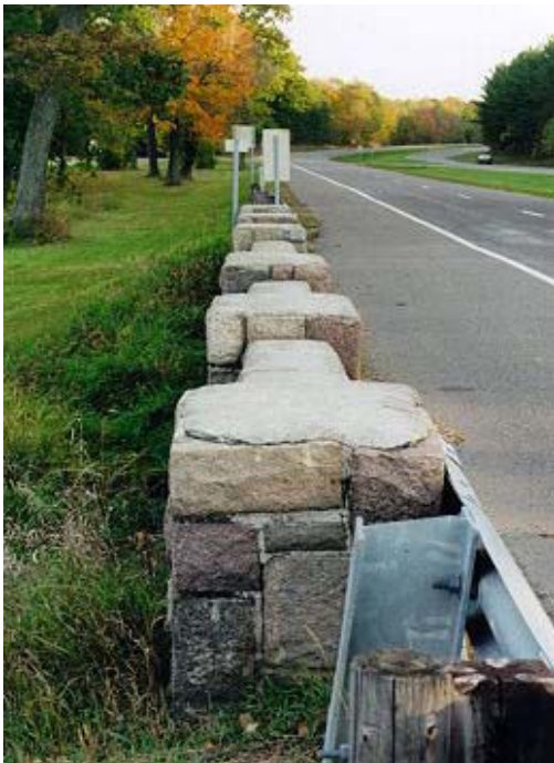
4. South End of Underpass looking North
