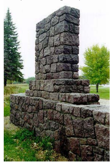
5. North View of Marker looking East
