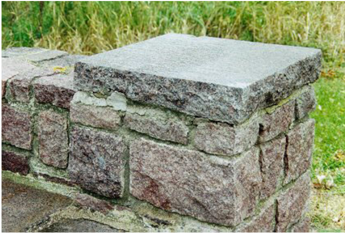
8. Close-up of Pier (Note: mortar patching)
