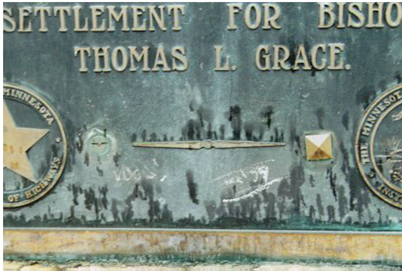
16. Bronze Plaque showing missing escutcheon and staining
