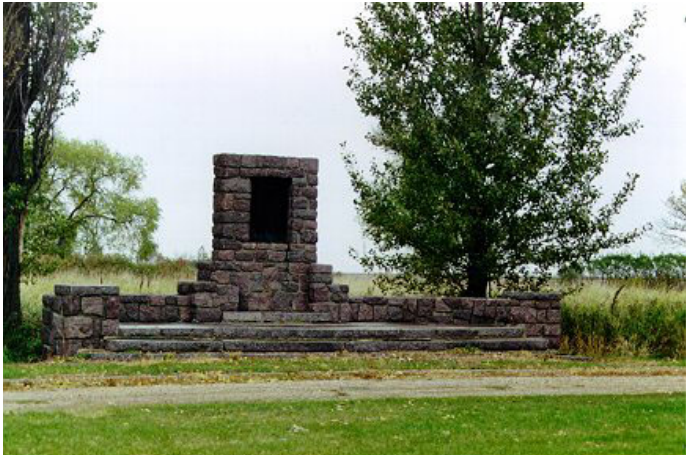
1. South Elevation looking North
