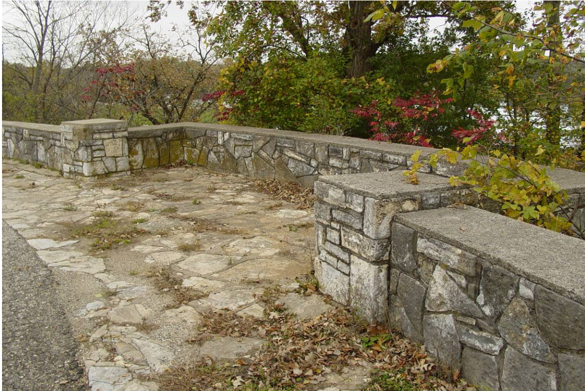
Plate 6. Overlook wall and flagstone terrace, facing southeast
