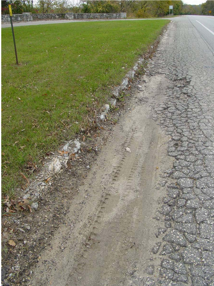
Plate 18. Stone curbing adjacent to TH 52, facing west
