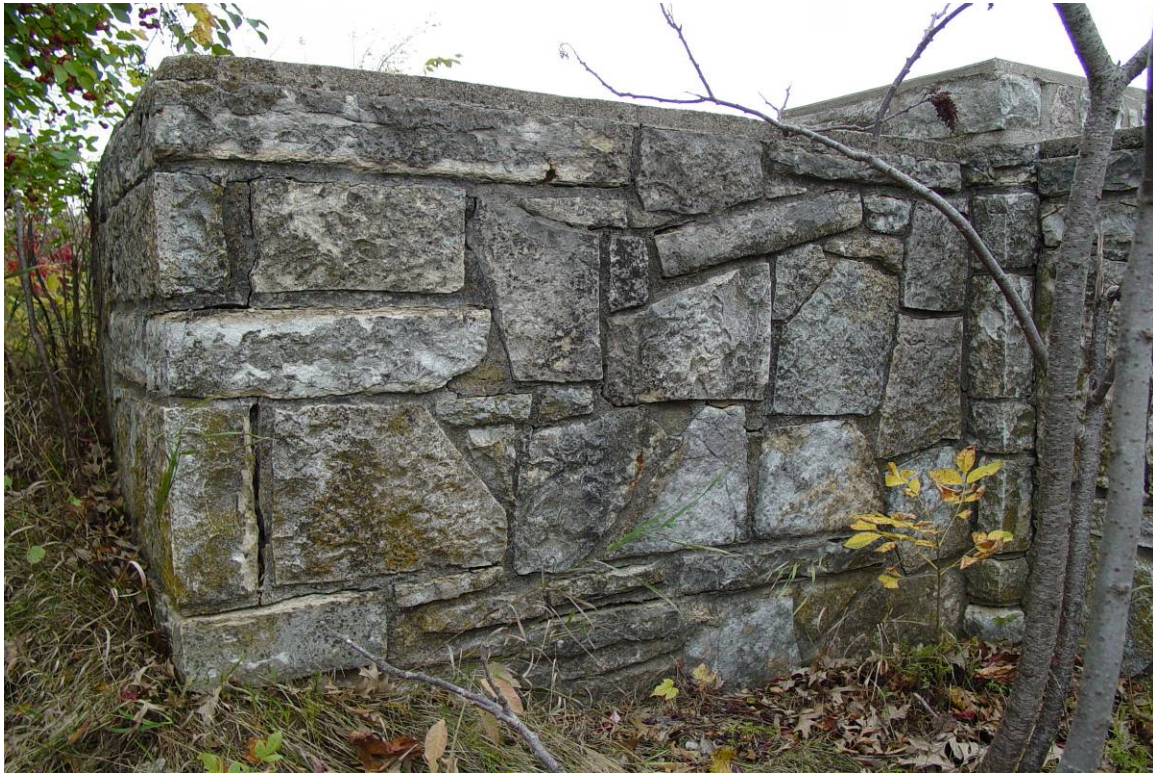
Plate 4. Outer façade near west end overlook wall, facing northwest
