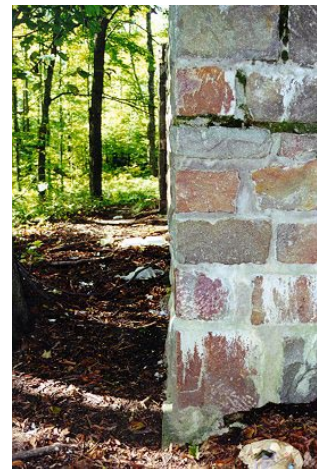
20. Recent mortar repairs.
