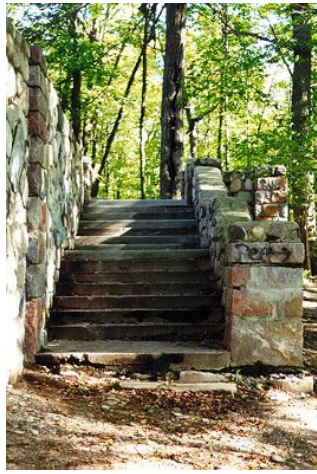
14. View new concrete step repairs.
