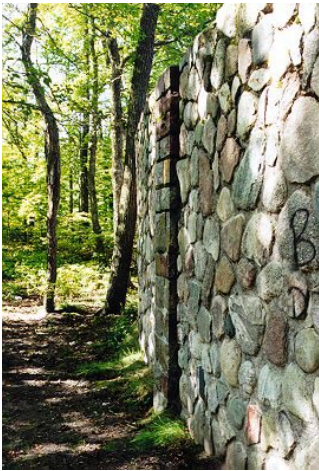
16. Base of overlook wall showing existing vegetation.
