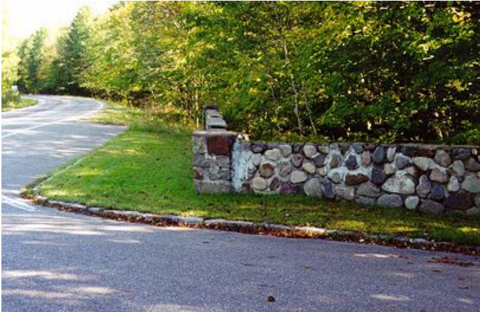
7. North site access – granite curb and stone wall (looking north).
