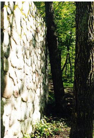
19. Lower wall view showing vegetation proximity.
