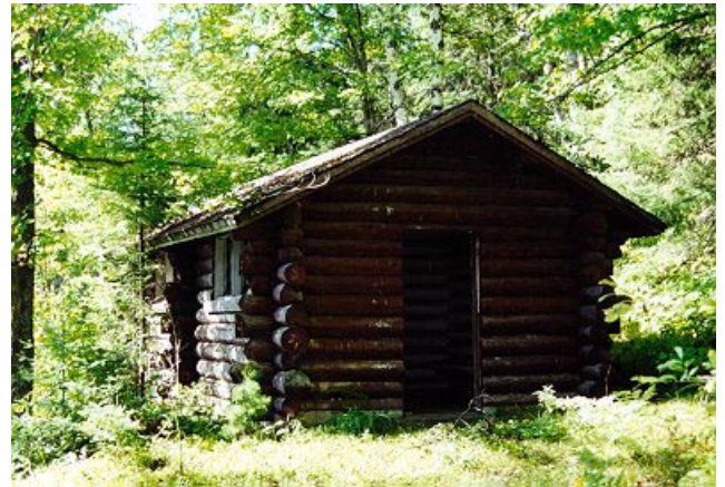
4. North east views of log bath house.
