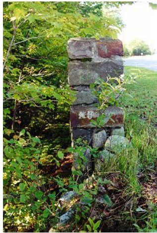
17. North end of overlook wall.
